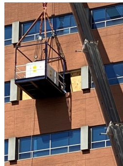
Signs outside the Leonard L. Williams Justice Center as an air handling unit is moved into place in April 2020.
